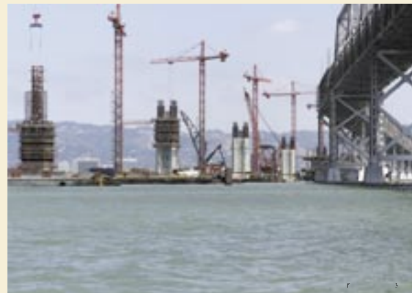
Bay Bridge Construction
